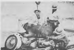
SOON AFTER his suggestion was accepted, Mechanical Department craftsmen began "hot tapping" the kerosene production line, left. PRONTO DESPUES cu su sugerencia a wordo aceptá, hendenan di Mechanical Department a cuminsa cu e trabao di "hot tap" ariba e linja di kerosene, robes.
